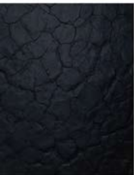
CYA8 crack size:1250*3100mm
